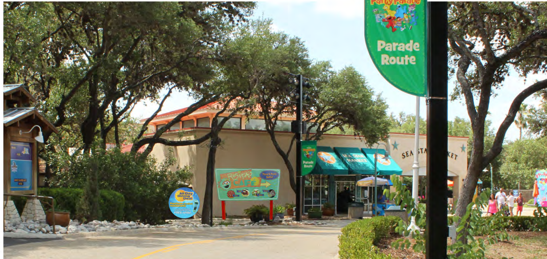
RELOCATE ROSITA'S CAFE SIGN TO POSITION SHOWN FOR VISIBILITY ON THE APPROACH
